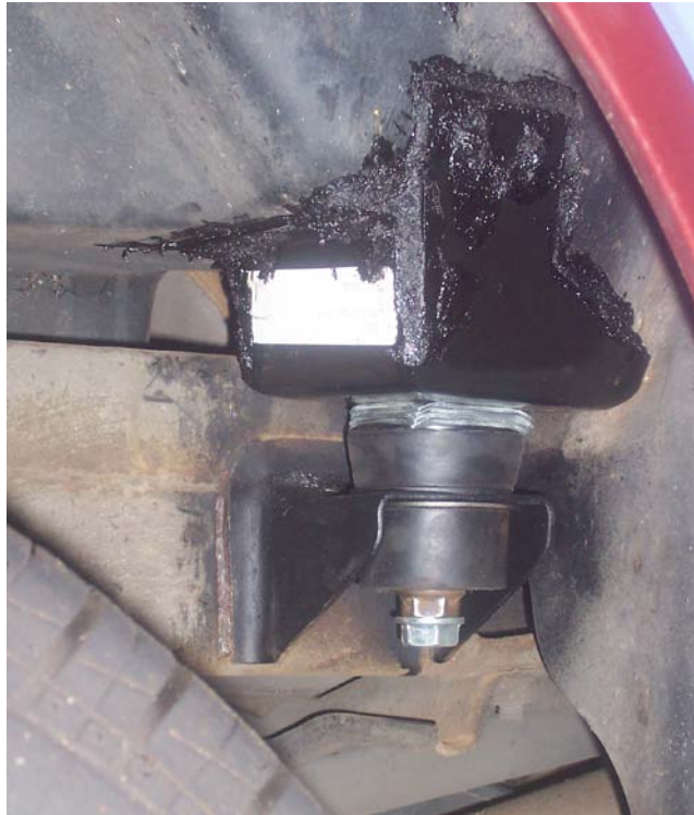
This is the new body mount and reinforcement installed in the left # 4 position.
