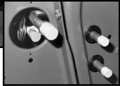
A/C and Heater Fittings Pass Through Existing Factory Holes In Firewall.
